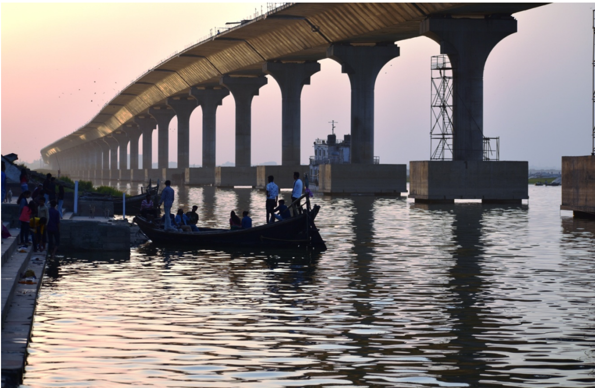
Image 2 : Ganga Expressway Under-Construction In River Along Ghats In Patna City
