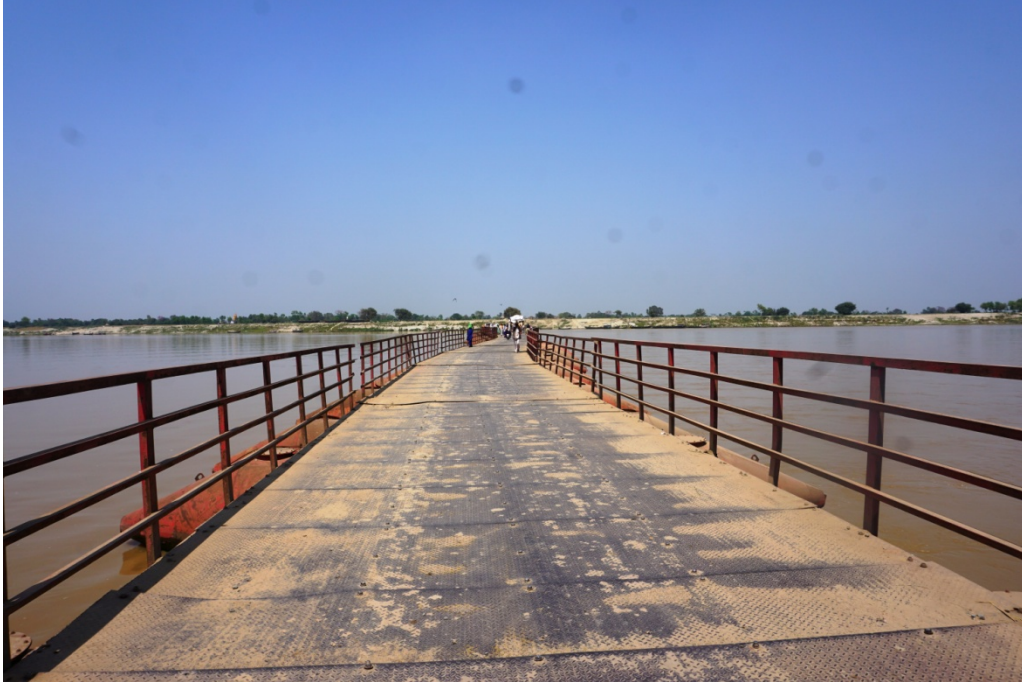
Image 20 : Pontoon Bridge Connecting RaghapurDiara With Patna Distt.
