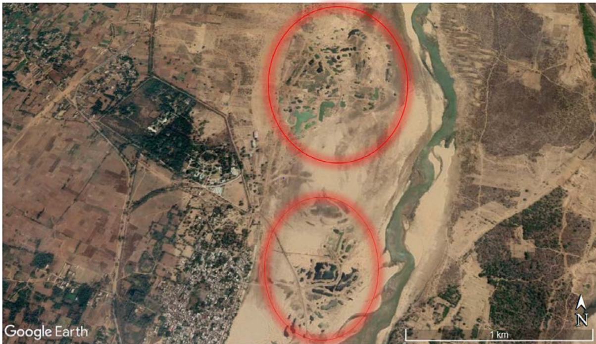
Image 5 : Satellite Image Showing Sand Mining In Son River Near Koilwar Rail Bridge
