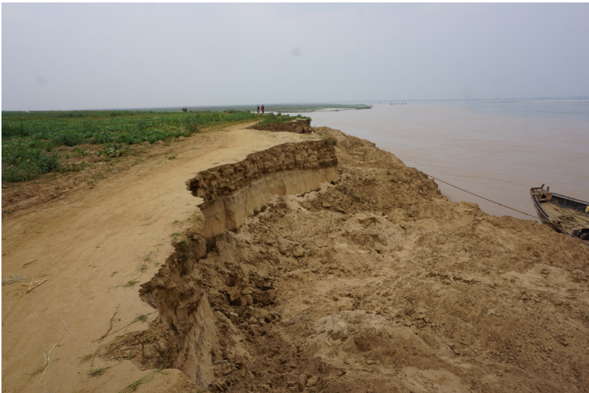
Image 30 : Eroded River Bank Near Haldichhapra Village [Right Bank]
